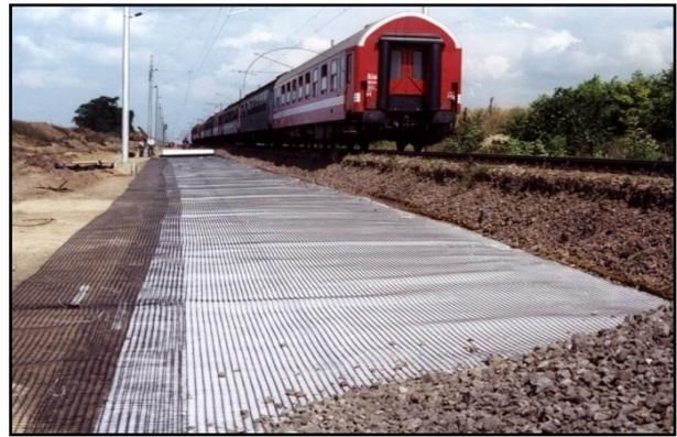
**Figure 2: Geogrid placed on geotextile directly on sub-grade soils awaiting sub-ballast installation, Bratislava to Trnava, Slovakia, 1999.**
