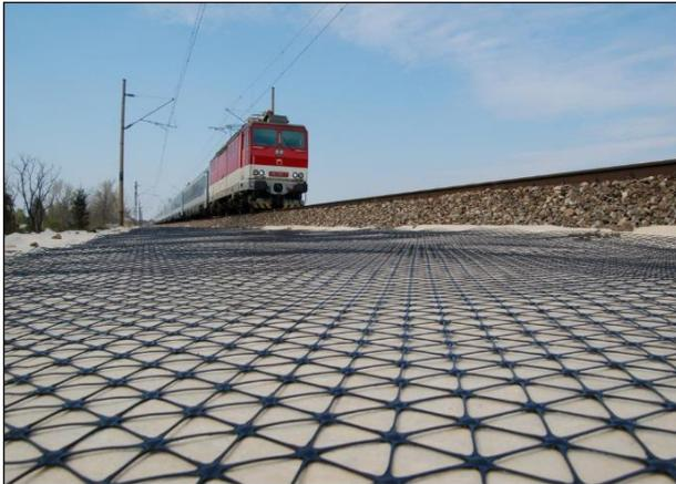
**Figure 11: Hexagonal stabilisation geogrid installed awaiting recycled sub-ballast, Bratislava, Slovakia.**
