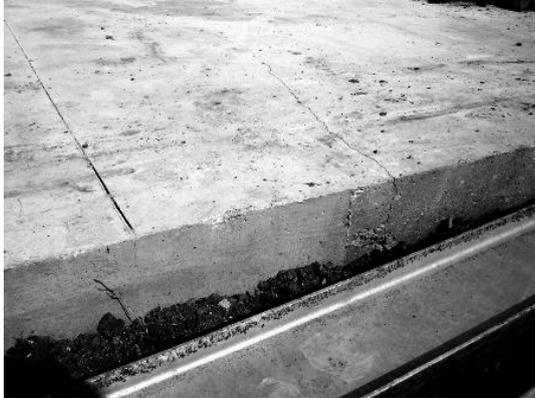
Cutting the groove too late could mean that the concrete will crack first
