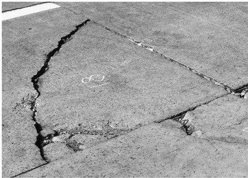
Severe faulting due to loss of load transfer capability in the crack
