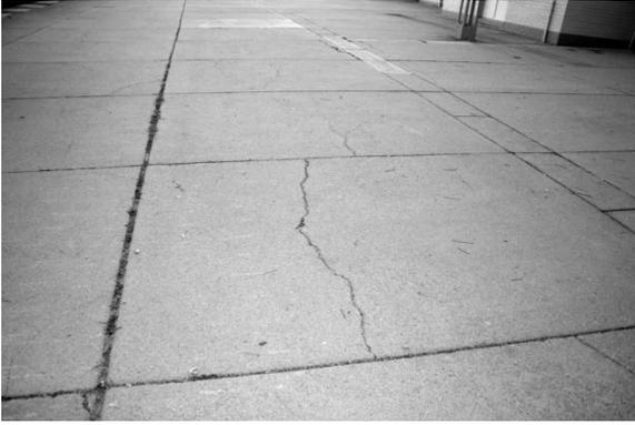
Typical drying shrinkage crack running across several panels of a pavement
